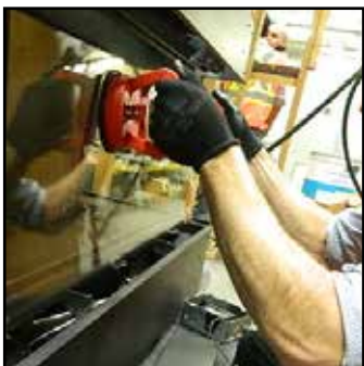
Handle glass with supplied vacuum clamps
