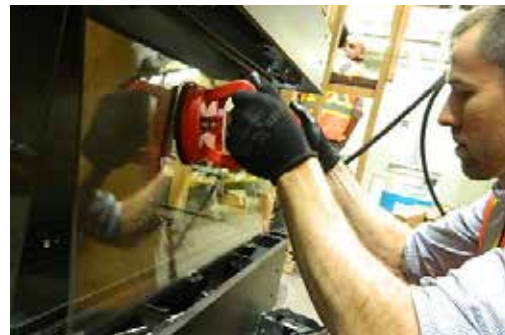
Handle front panel with supplied vacuum clamps
