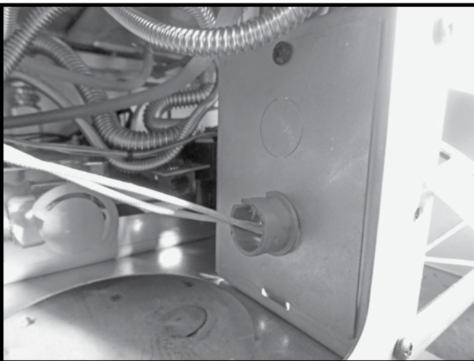
Figure 90: Threading wires through knockout.
