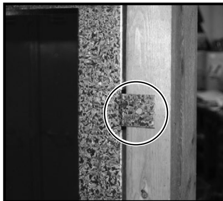
Figure 20: Attaching metal tab to frame.
