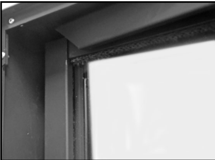
Figure 81: Installing top trim.
