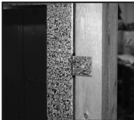
Figure 17: Attaching metal tab to frame.
