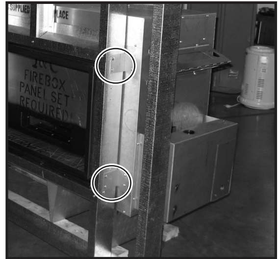
Figure 19: Framing bracket fastening points.
