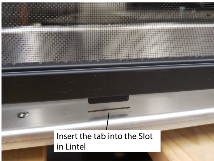
Figure 22: Screen Tab install.ai
