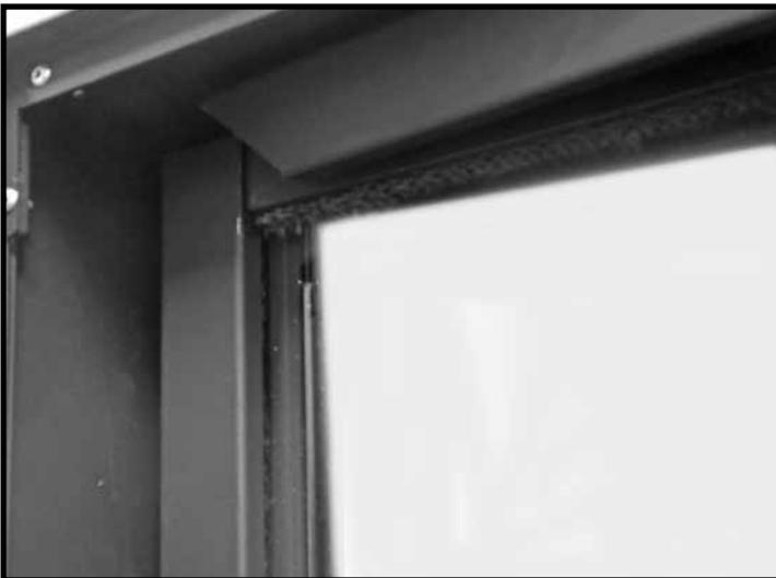
Figure 57: Installing top trim.
