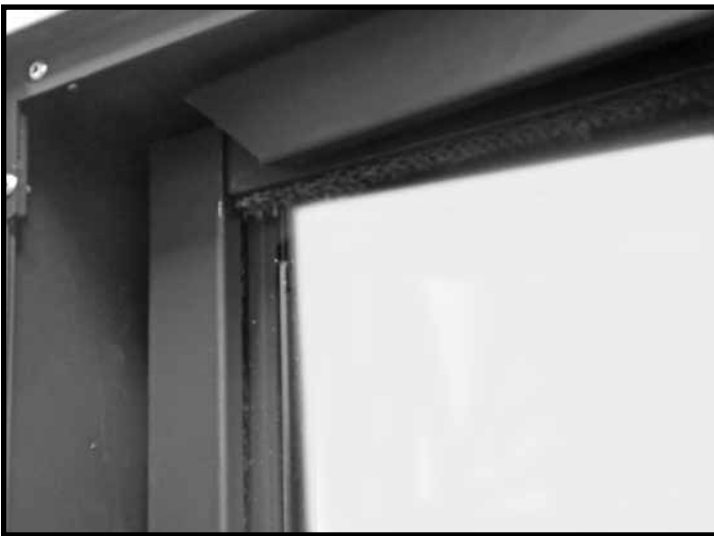
Figure 57: Installing top trim.
