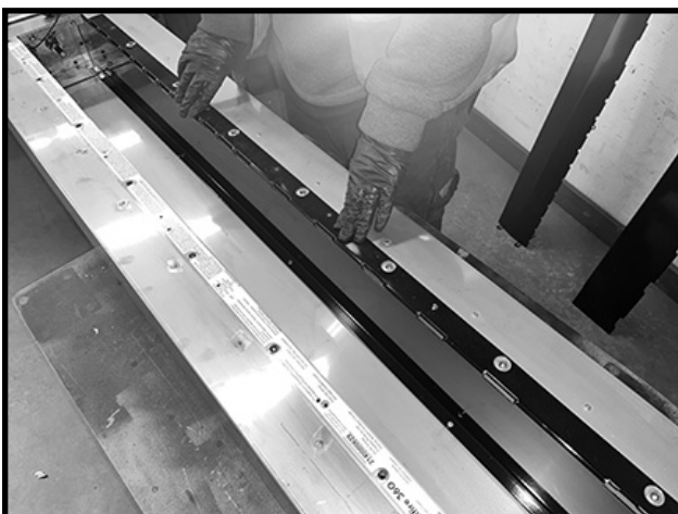
Figure 40: Reinstall double flanged panel.
