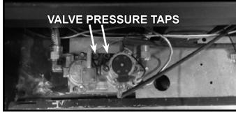
Figure 9.1 Valve Pressure Taps
