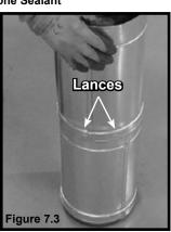
**Note:** Make sure that the seams are not aligned to prevent unintentional disconnection.
