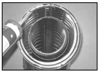
Figure 7.1 High Temperature Silicone Sealant
