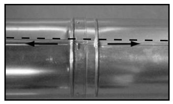
Figure 7.10 Align and Disassemble Vent Sections
