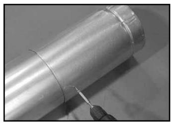
Figure 7.6 Screws into Slip Section
