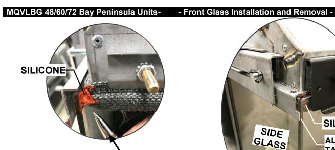
**⚠ IMPORTANT:** Each corner must have a dab of high-temp silicone placed between the ball of the gasket and the corner glass. This will fully seal the firebox corners.
