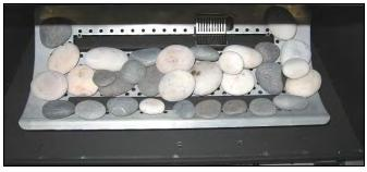
Place smaller stones around outside of burner tube.
