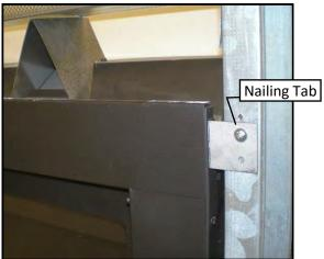
**Step 2:** Use concrete board to cover face of fireplace. **NOTE:** Leave clearance of 1-3/16" on top and 1-1/16" on both sides and bottom to install and remove screen.
