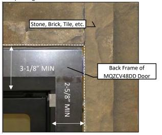
**Step Two:** Use Drywall to finish face of wall. **NOTE:** Wall will be flush with fireplace face.
